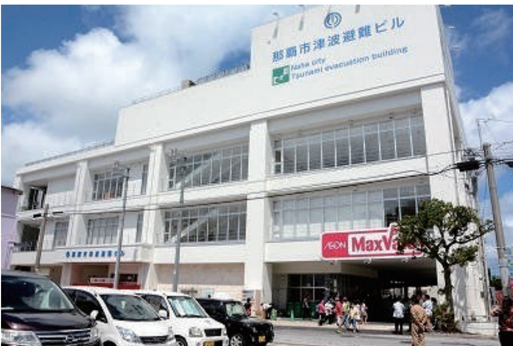
Naha city Tsunami Evacuation Building (2-22-1 Matsuyama Naha city)
